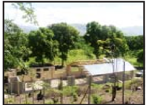
New church under construction on higher ground in Sous Raille.
